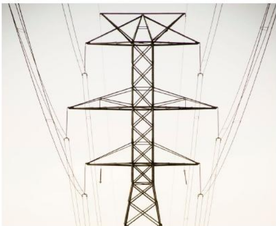
Figure 3: A Transmission Tower
