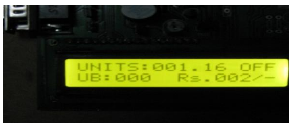
Fig.10: LCD showing the power consumption values and the billed amount and status of the system is also displayed when it is OFF.
