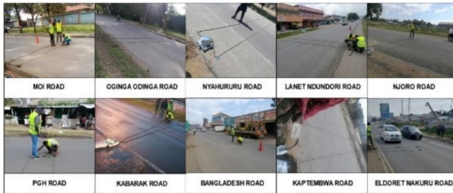
[Fig.2: Installation of Metro Count Roadside Units on Site]
