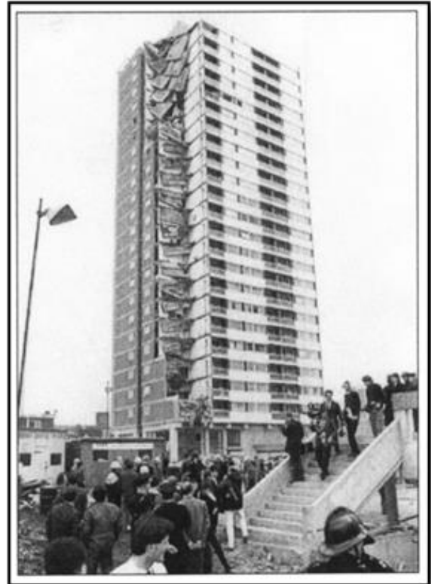
Figure 1. Ronan Point apartment building after the collapse [16]
