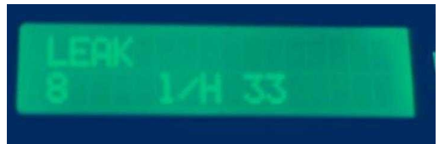
Fig. 10: Display that water leaks from the pipe
