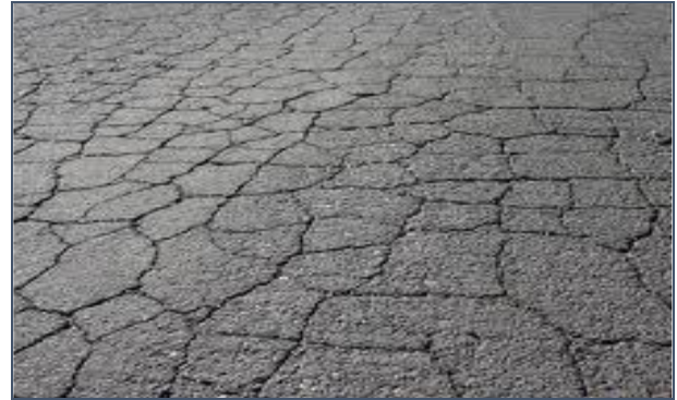
Figure 5: Fatigue cracking [51]
