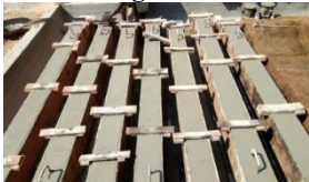
Fig. 4 Beams after Casting
