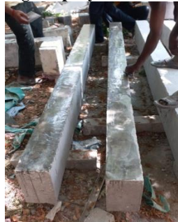
Fig. 9 Application of Epoxy Resin
