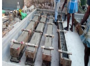
Fig. 3 Concrete being Placed and Compacted
