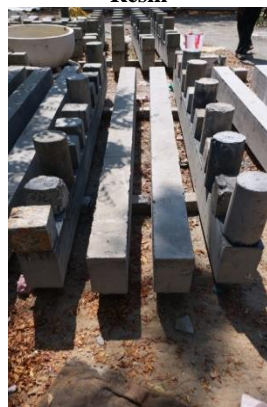
Fig. 11 Placing of Weight over the Laminate
