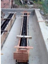
Fig. 2 Wooden Mould for Casting of Beams
