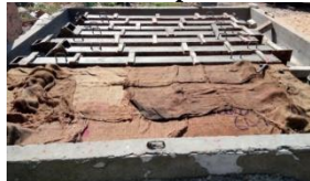
Fig. 5 Beams under Curing
