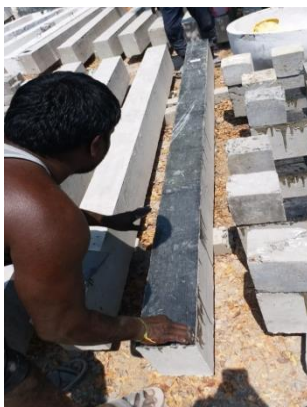
Fig. 10 Placement of HyFRP
